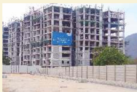
Access Road - Work-in-progress
