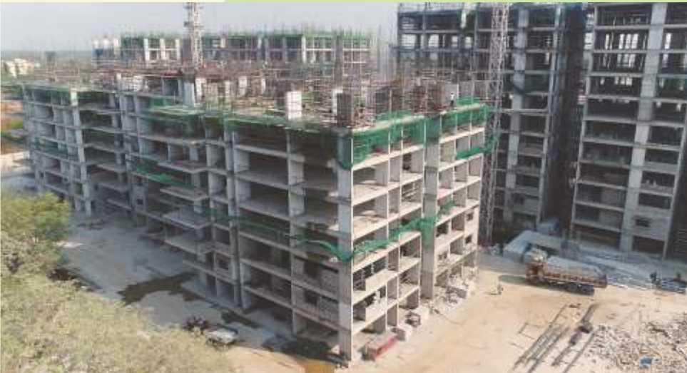
Kailash North-west View - 7th Floor
