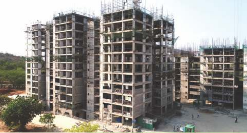
Everest East View - 11th Floor
