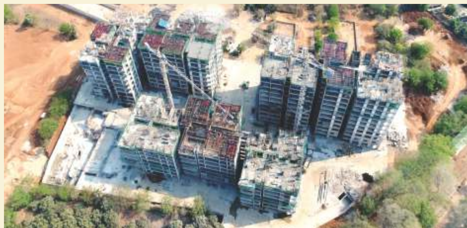
Top View from North Side
