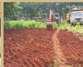
REMOVAL OF TOP SOIL
