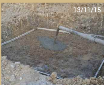
FOUNDATION WORKS STARTING
