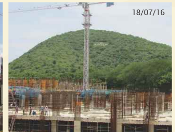
KAILASH - B-1 LEVEL SLAB
