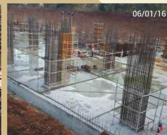
COMPLETION OF RAFT FOUNDATION
